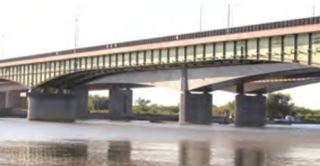
Bridges in Kiezmark. Photo: R. Wasil
