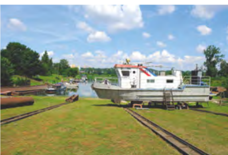
The shipyard slipway in Gorzów Wielkopolski. Photo: Berda.pl
