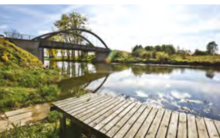
The Osiek Bridge over the Noteć River. Photo: P. Pasieczny
