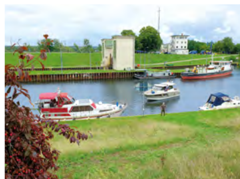
Locks at Hohensaaten. Photo: Berda.pl
