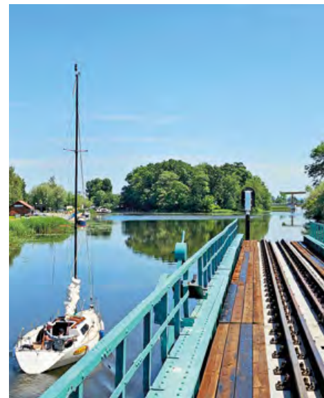
View from the railway bridge of the Szkarpała. Photo: R. Wasil
