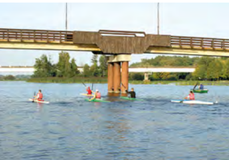
"St. Adalbert" pedestrian bridge Photo: P. Salecki
