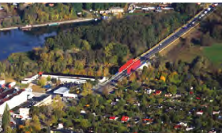
Railway bridge of the Coal Trunk Line. Fot. M. Szelest
