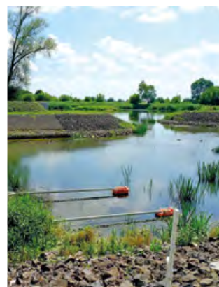
Entrance to the marina basin. Photo: Berda.pl
