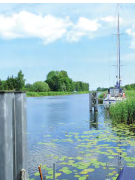
Guide dolphins of the drawbridge in Drownica Photo: Berda.pl
