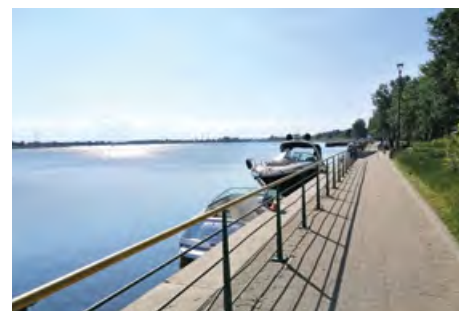
Mooring quay in Sobieszewo. Photo: R. Wasil
