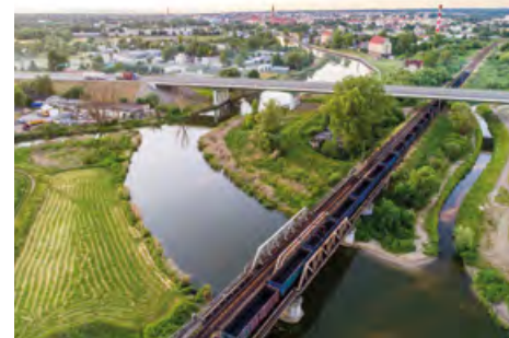
The Elbląg River. The S7 expressway bridge and the railway bridge. Photo: A. Wołosz
